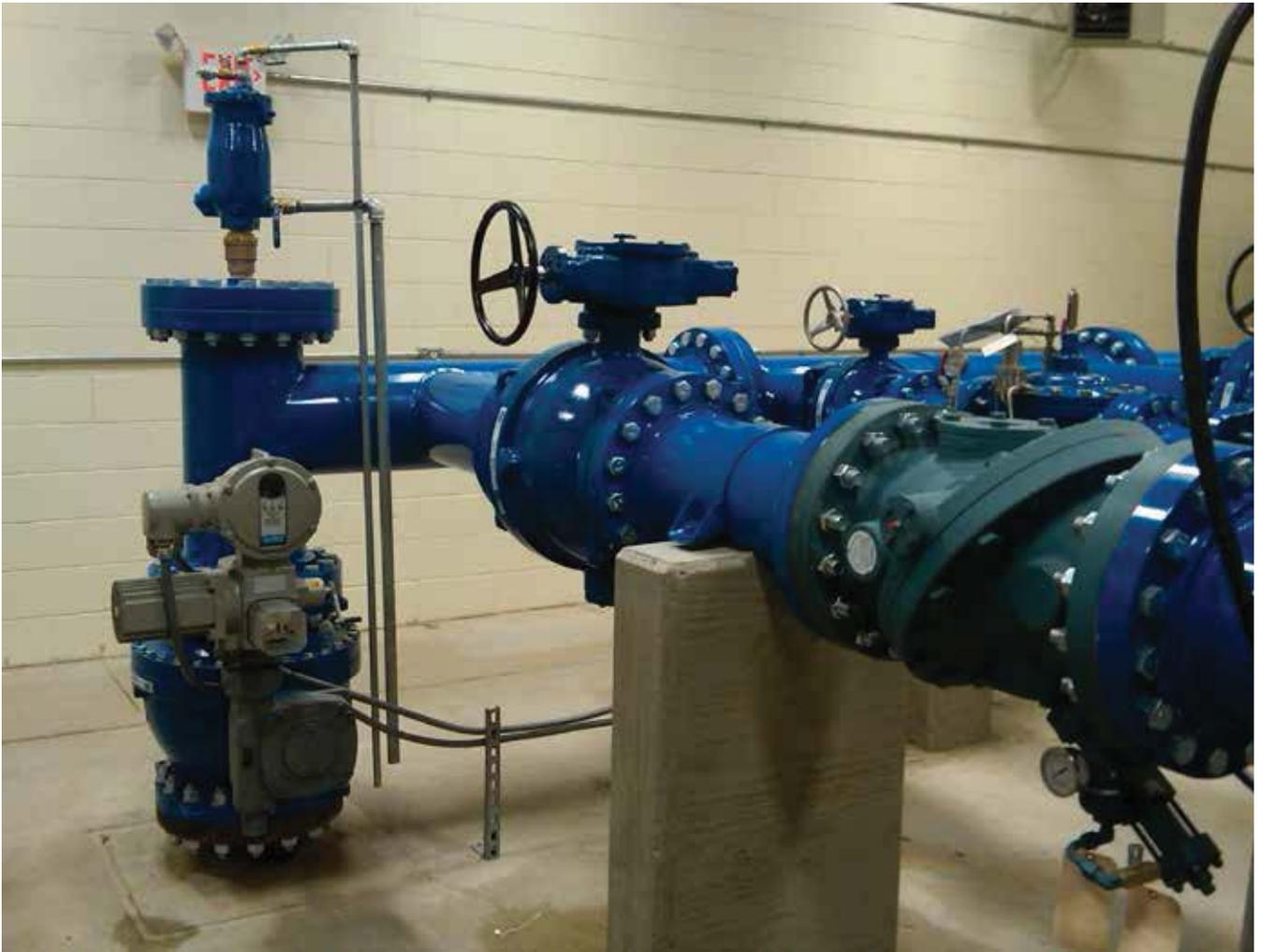
A VSA actuator bridges the gap between theory and reality for control of pressure surges
