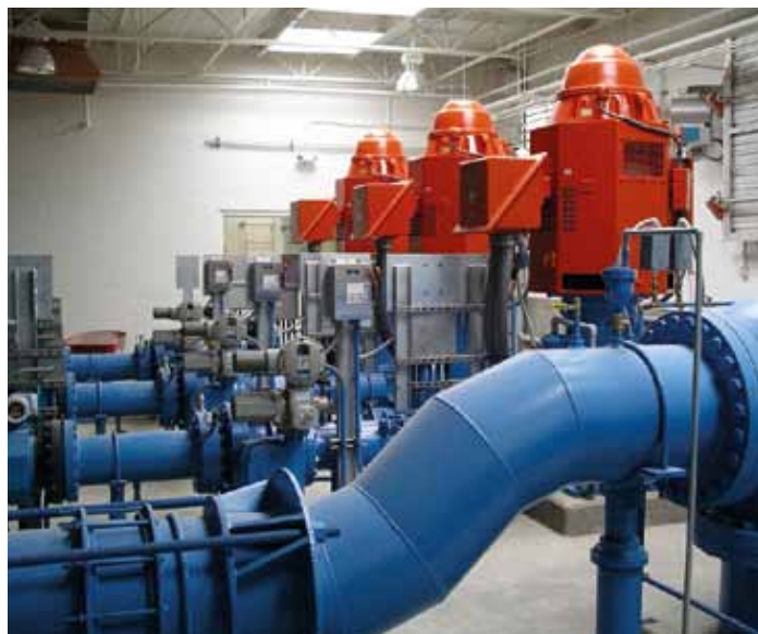
SIPOS Aktorik actuators address water hammer at ECCV pump station.
