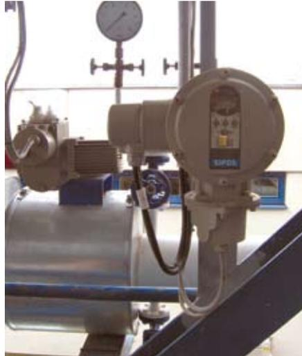
Actuators from SIPOS Aktorik stabilize the control circuits in the waste-fuelled CHP
