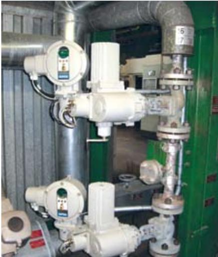
SIPOS actuators with integral frequency converters installed at Rosenheim
