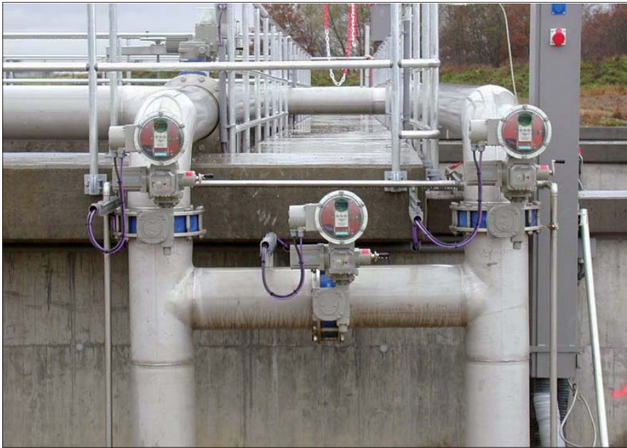
Fig. 4: SIPOS actuators – despite exposure to all kinds of weather, these 2SC5 part-turn actuators always supply and discharge reliably
