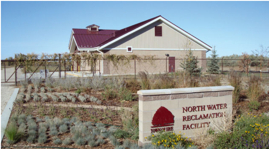
North Water Reclamation Facility
