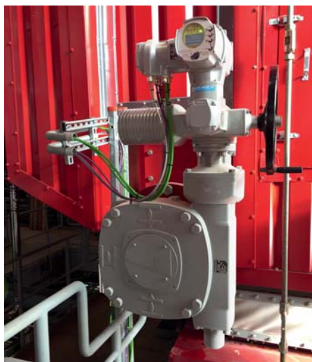
An AUMA SA 14.6 actuator with AC 01.2 SIL actuator controls and GS 250.3 gearbox meets SIL 2 requirements for the condenser bypass damper at Lisbjerg power plant.
