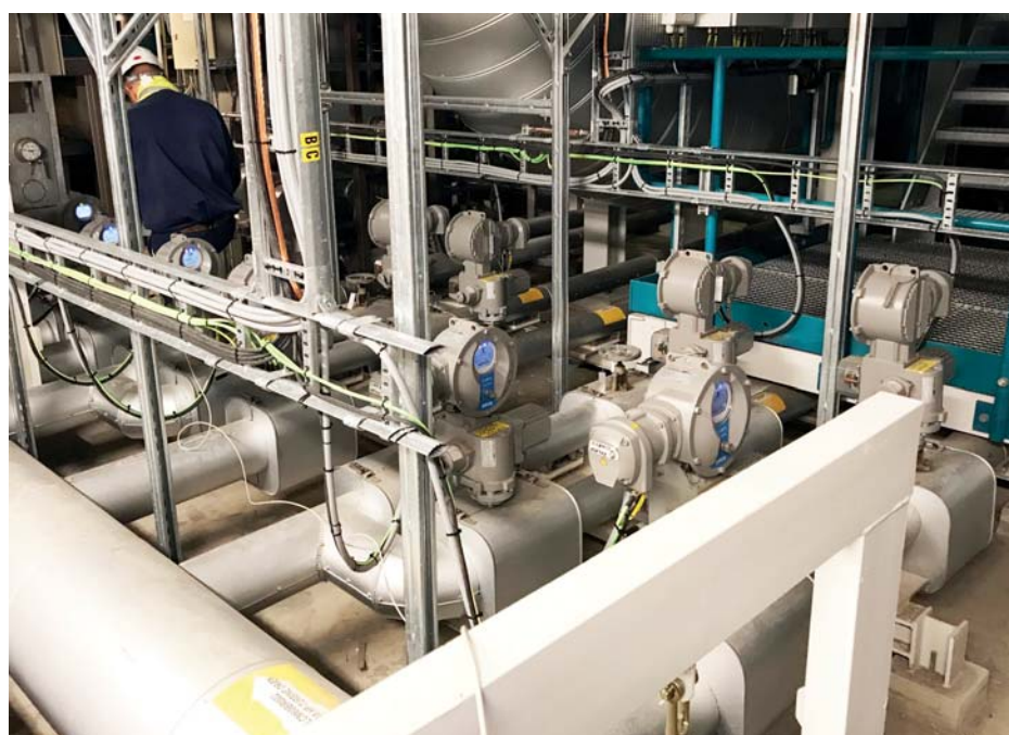
SIPOS SEVEN actuators with Profibus DP interface (V2 services as standard) in Skærbæk power plant.
