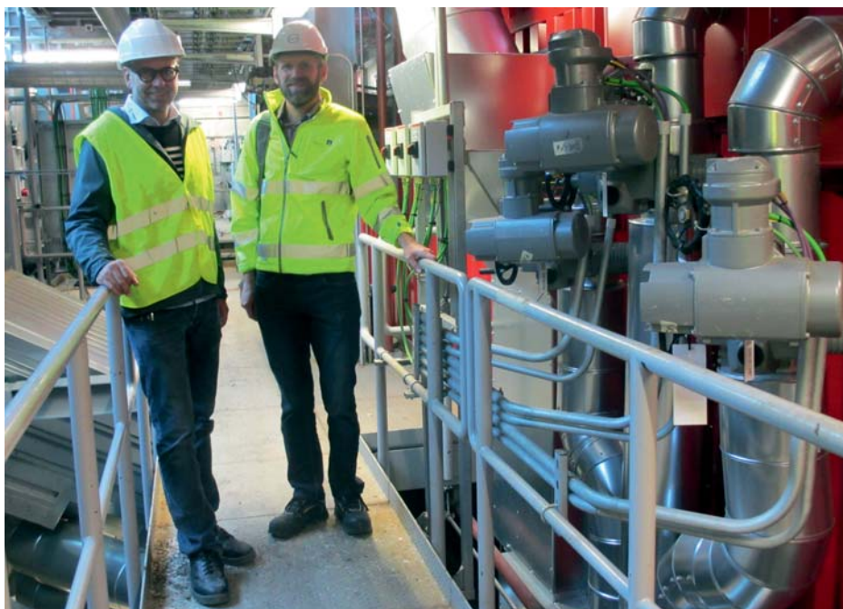
AUMA's modular SA and SQ electric actuators control the flow of water and steam at Lisbjerg power plant.
