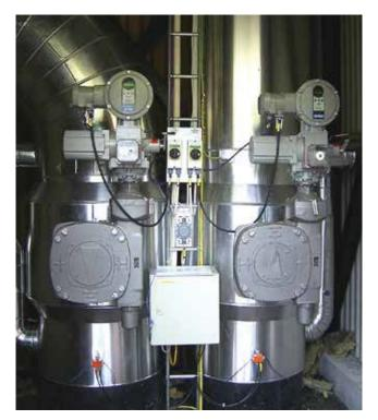
Variable Speed Actuation technology addresses water hammer
