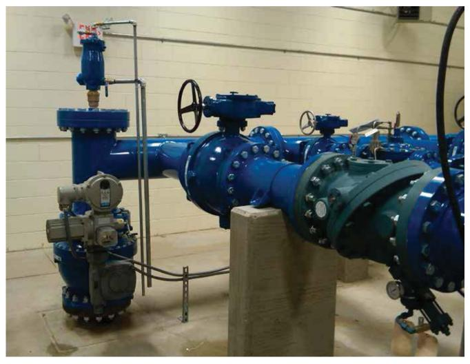
A VSA actuator bridges the gap between theory and reality for control of pressure surges
