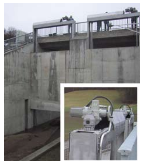
VSAs – a new force in flood applications (photograph of Brettachtal basin installation)
