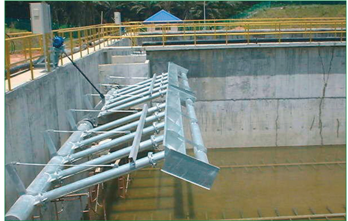
Fig. 7: Variable speed actuator system on a decanter in a sewage treatment plant
