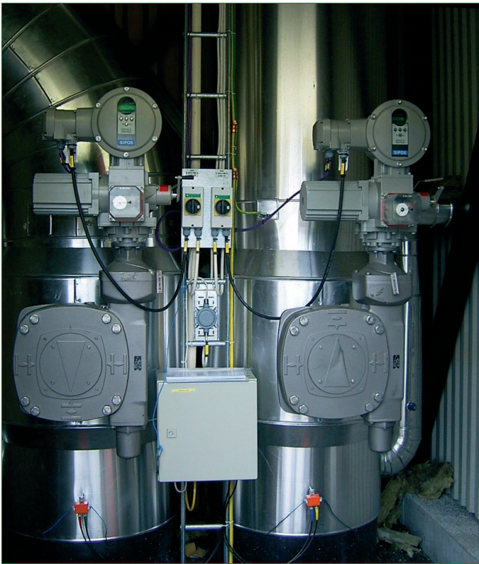
Fig. 10: SIPOS 5 Flash in a district heating pumping station
