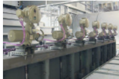
Redundant fieldbus control in a large power plant
